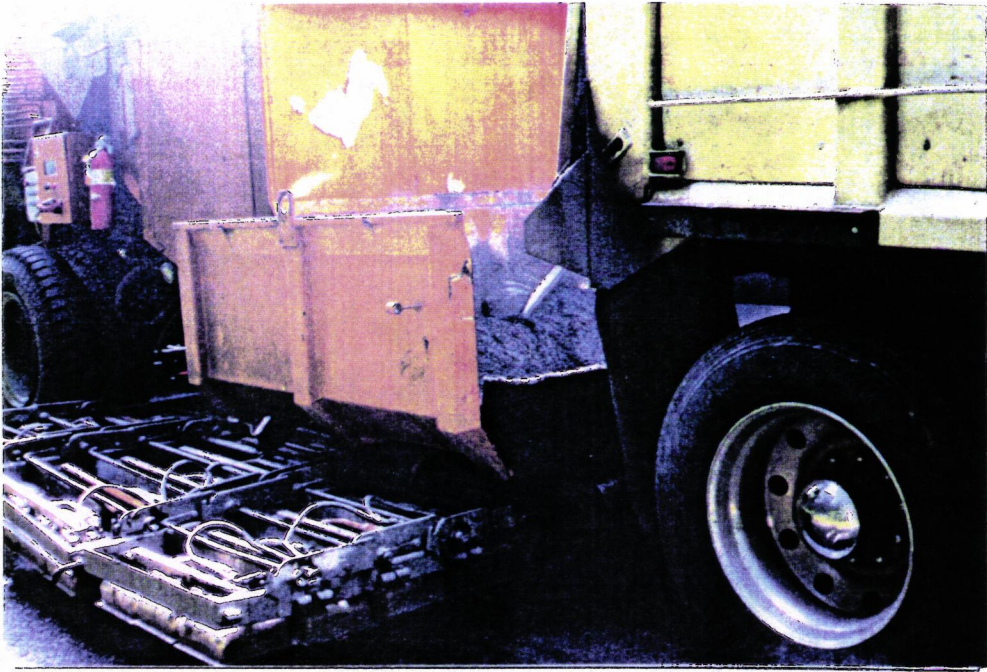
Virgin Hot Mix is Delivered to Receiving Hopper
