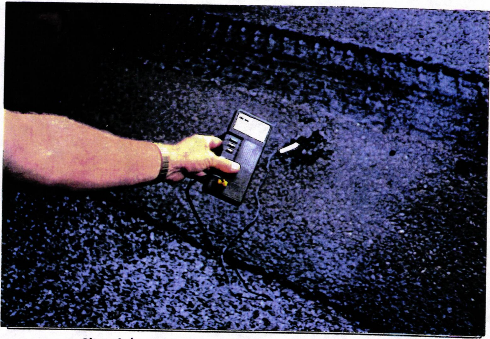
Checking Temperature of Recycled Mat
