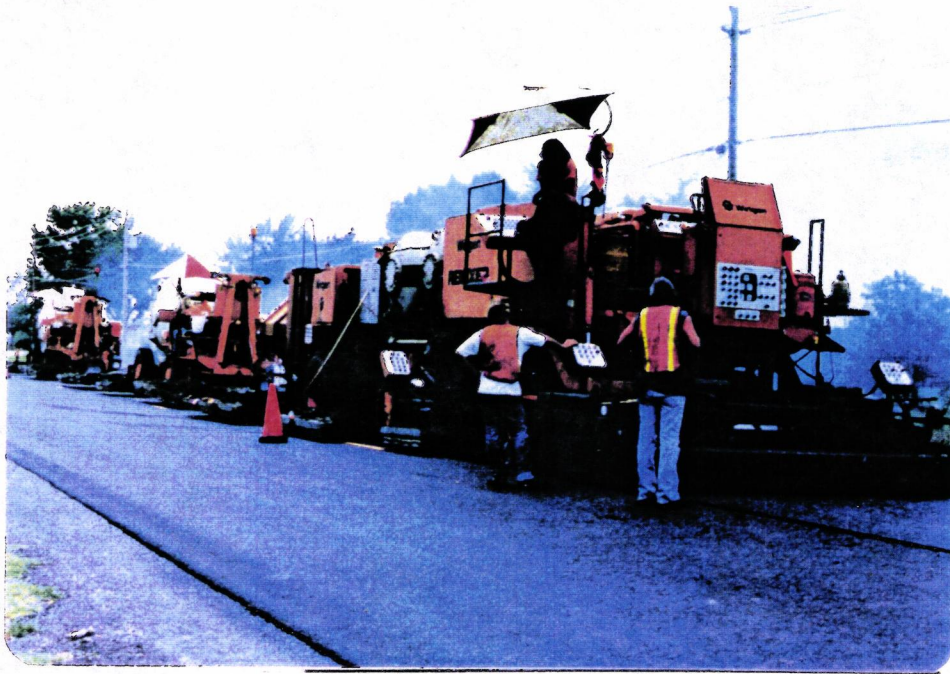
View of In-Place Recycling Operation
