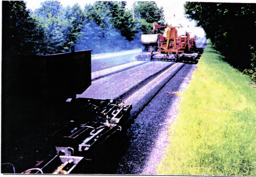
View from Hopper Back to Heating Panels
