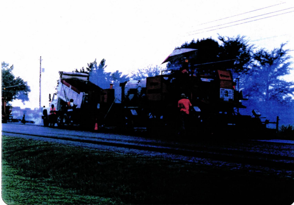
Paver Pauses as New Hot Mix is Delivered
