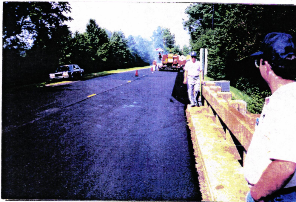
View of New In-Place Recycled Surface
