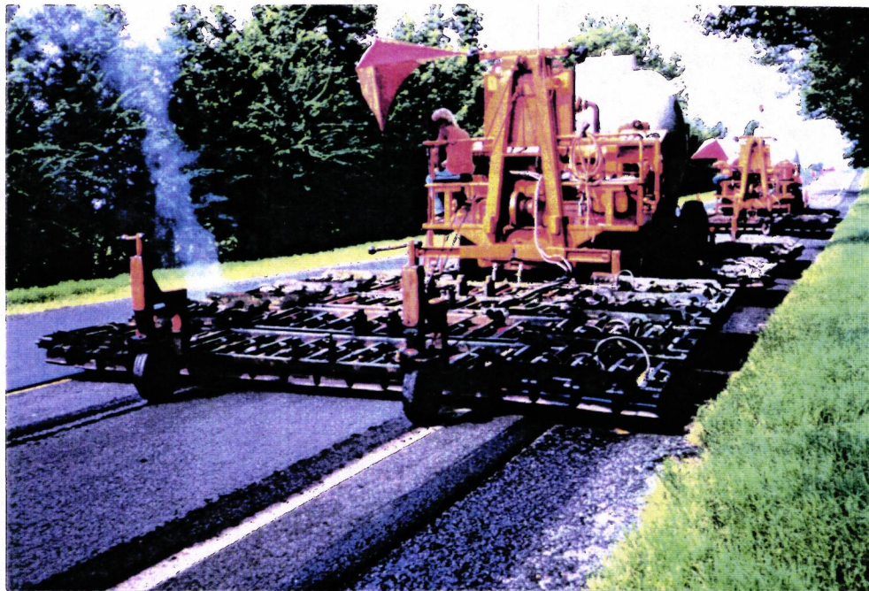
Infra-red Panels Preheat Pavement
