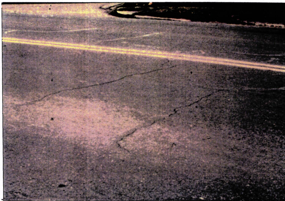
Texarkana Bad Test Section (3 years after const.)
