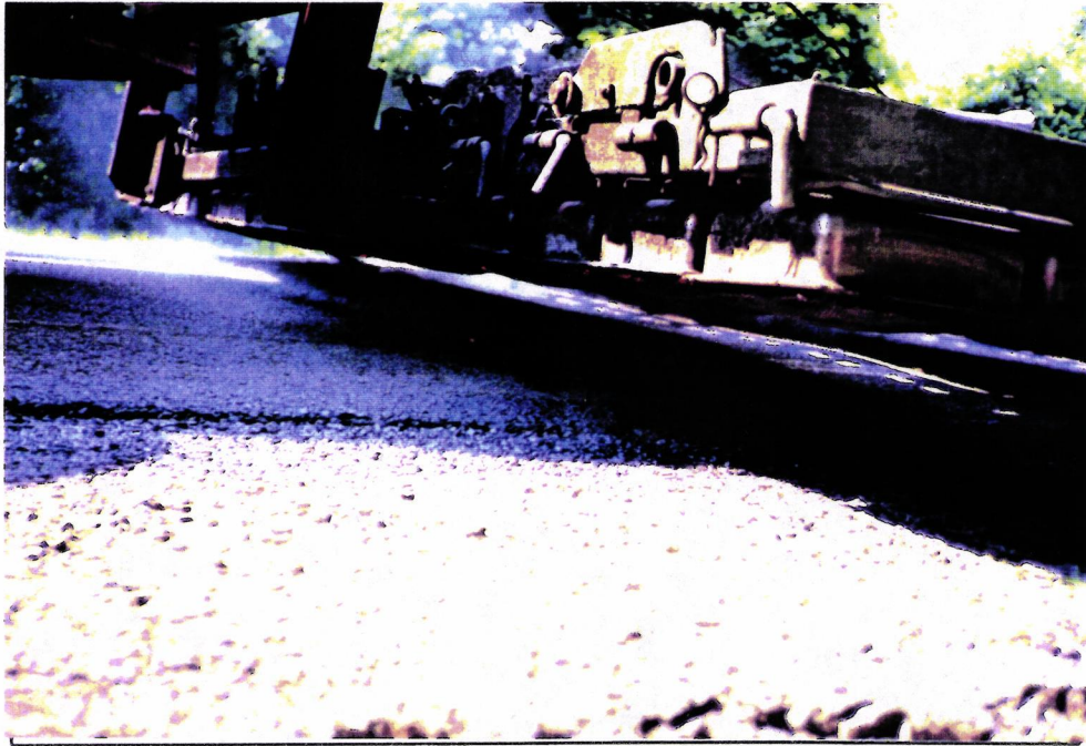
Infra-red Panels Heating Existing Pavement
